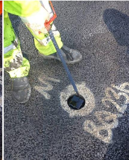
Although these units were installed whilst the sections of road were closed, it proved that they can be fitted in a much quicker time than a traditional inductive loop, and that because they are positioned in the centre
