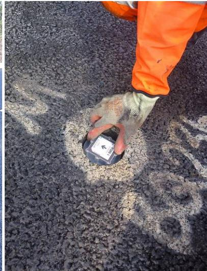
Unit sealed in place with epoxy resin
